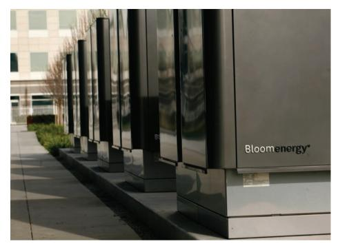
▲ Figure 1.20 Solid-State fuel cells manufactured by Bloom Energy.
